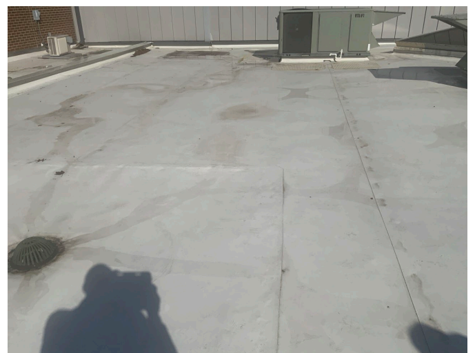
6 - PVC/TPO MEMBRANE ROOFING
