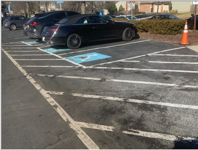
OVERVIEW OF ACCESSIBLE PARKING AREA
