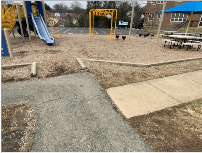
ACCESSIBLE ROUTE TO PLAYGROUND
