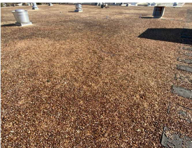
5 - BUILT UP ROOFING
